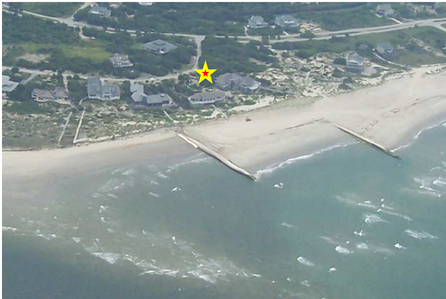
3. July 7, 2011 Following Emergency Repair to Groin #16
