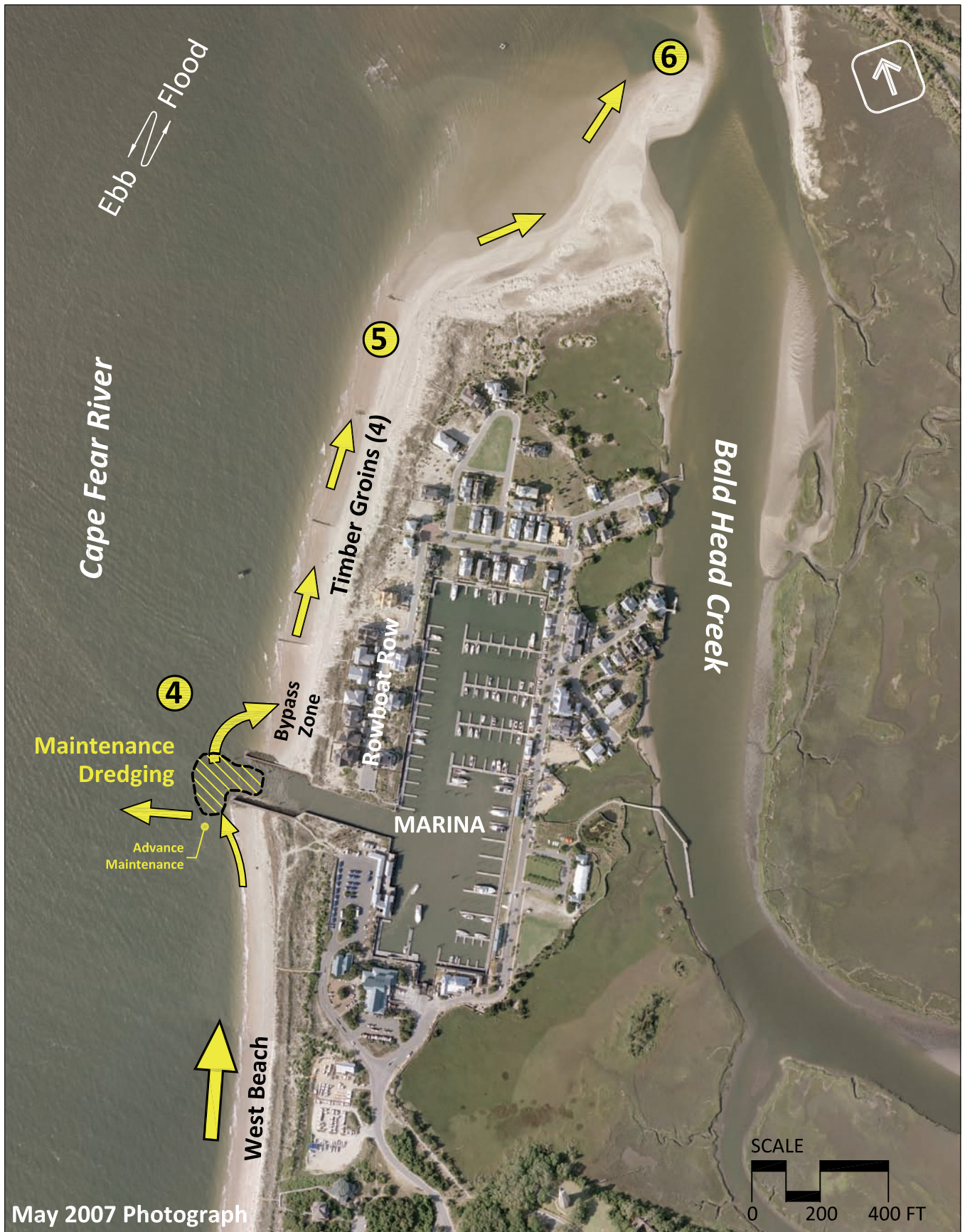
Figure 2: Sediment transport bypass trends at the marina entrance (West Beach).
